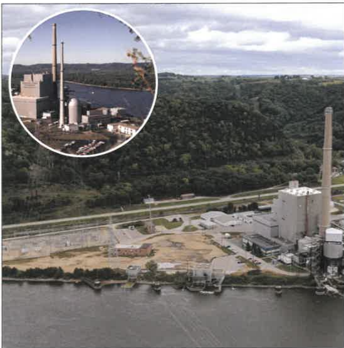
^ Located on the banks of the Mississippi River, the La Crosse Boiling Water Reactor has been successfully decommissioned, the land fully restored, and final approval to transfer the license back to Dairyland Power Cooperative is expected in 2022.
