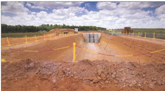
^ Disposal trench for containerized waste at Barnwell disposal facility.
