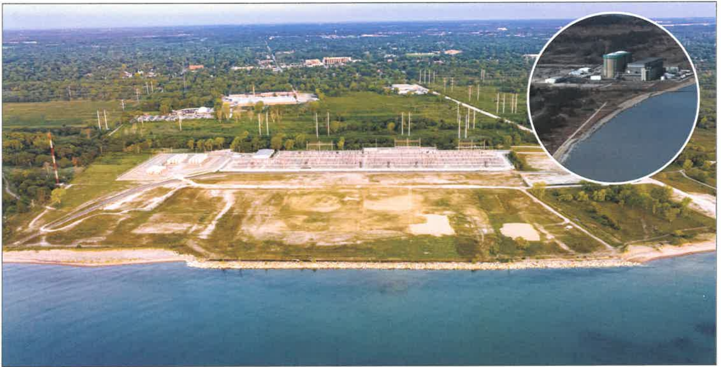
^ The decommissioning of the Zion power plant advanced the restoration of the Lake Michigan property to its natural state by nearly thirty years. The project set world records for the largest and most successful spent fuel transfer campaign, as well as the most cost-effective reactor vessel internals segmentation project to date.
