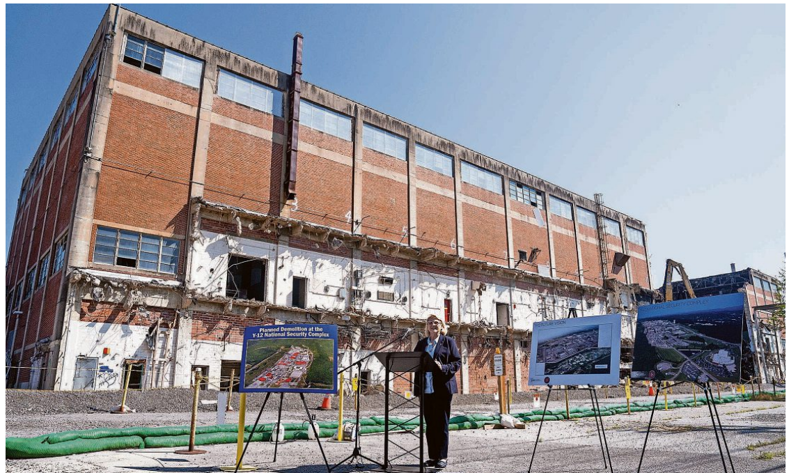
Susan Morris, deputy manager of the National Nuclear Security Administration – Y-12 office, speaks to the media as demolition of the Alpha-2 Complex continues at the Y-12 National Security Complex in Oak Ridge on July 8. The complex was built for uranium enrichment operations as part of the Manhattan Project and once housed the equipment monitored by the famous "Calutron Girls." BRIANNA PACIORKA/NEWS SENTINEL
