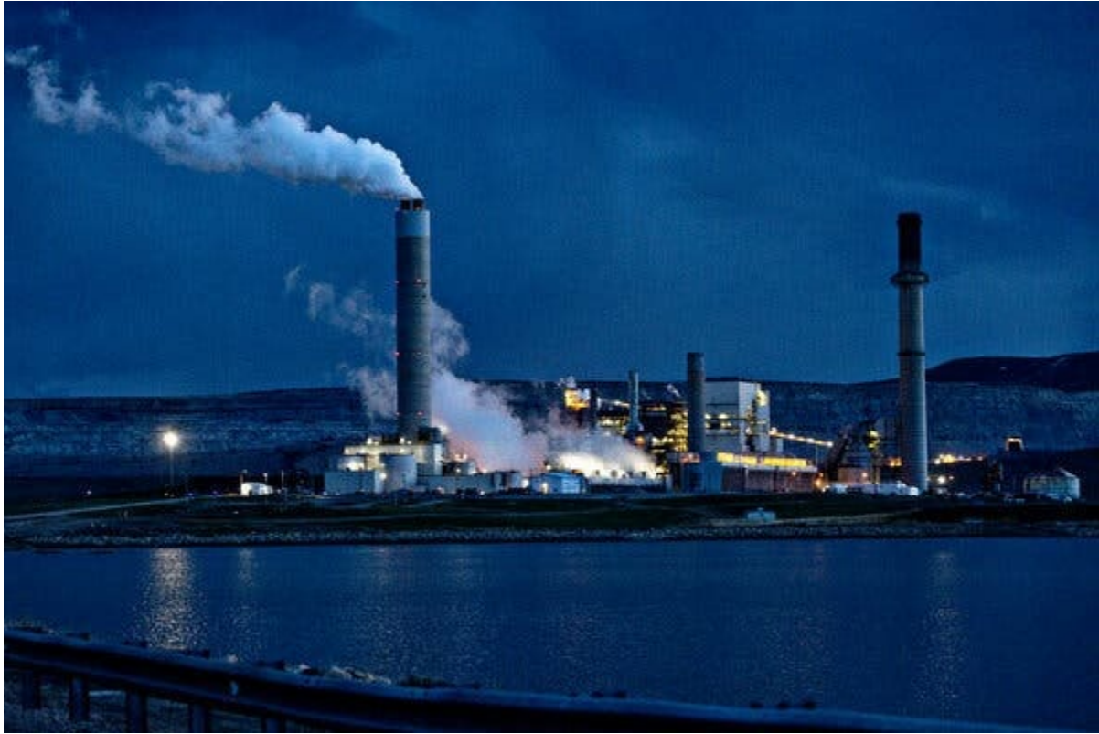
The Naughton coal plant, outside Kemmerer, is set to be decommissioned in 2025. Credit...Kim Raff for The New York Times
